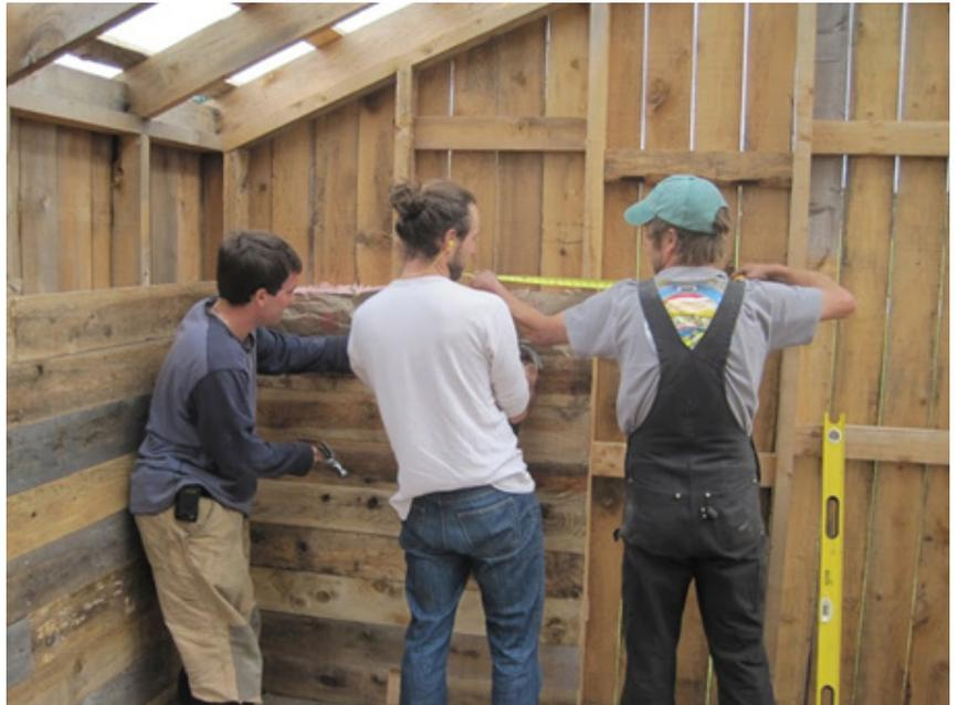
*Figure 3: Building the insulated bin walls*
