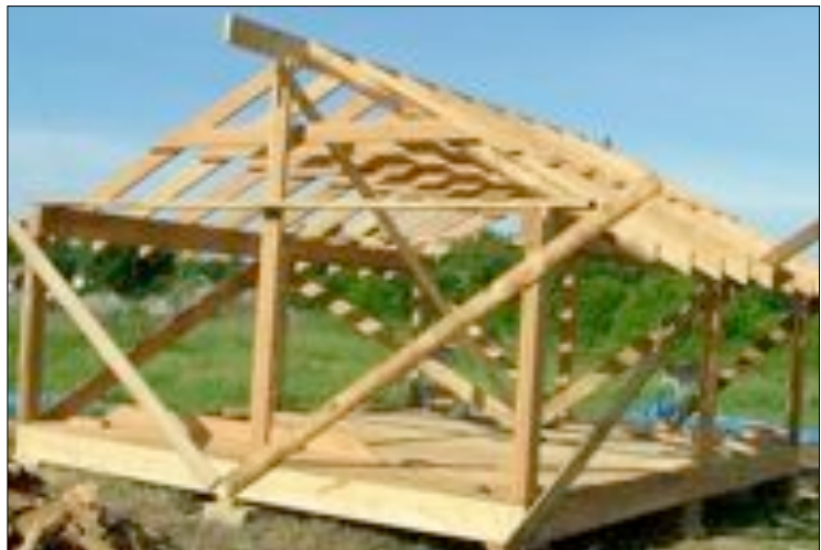
Enclosed composting system for Ferrisburgh Central School under construction
